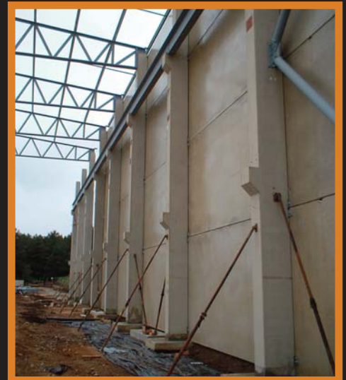
Columns & Retaining Units
