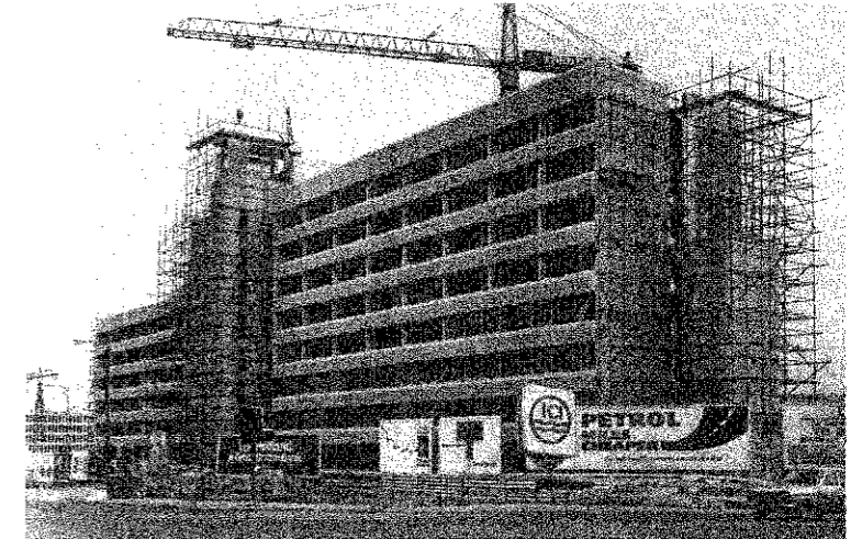
T6 multi-storey framework, Bradford.
