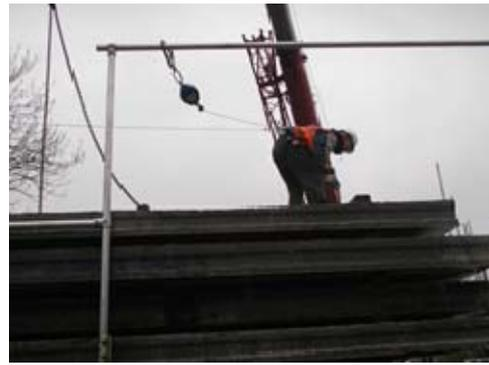
If the load is two stacks, the slinger is attached to one inertia reel at a time. Once the first stack has been offloaded, the slinger then switches inertia reels so that offloading of the second stack can commence.
